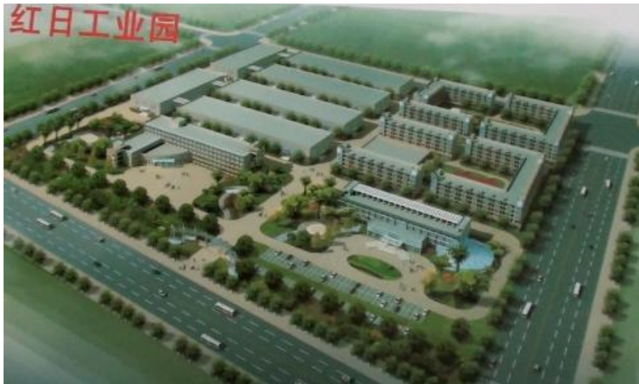
KBS's planned manufacturing plant 2011/2012
